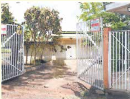
The Central Radio Waste Management Facility (CRWMF) in Arusha
